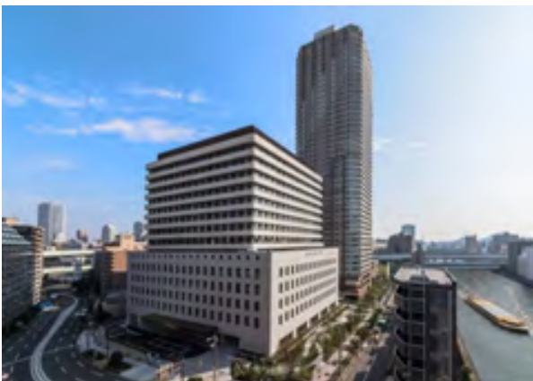
Exterior of Nippon Life Hospital
